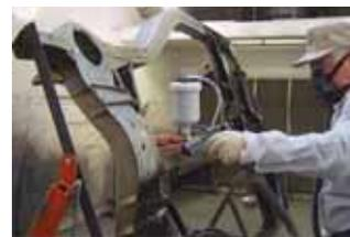
**Frame Painting** - Darney rolled out his TP Tools HVLP Turbine System with Gravity Gun to apply three coats of POR-15<sup>®</sup> Semi-Gloss Rust Preventive Paint to seal and protect the new frame. Later, he applied two coats of POR-15<sup>®</sup> Chassis Coat Black<sup>™</sup> Topcoat Paint to
